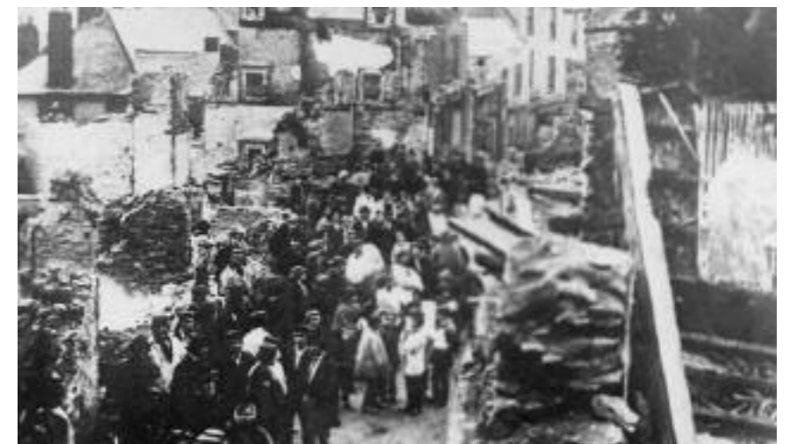
Aftermath of the High Street Fire
