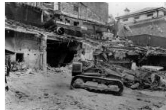
Demolition of The Classic to make way for Tesco's, Summer 1970
